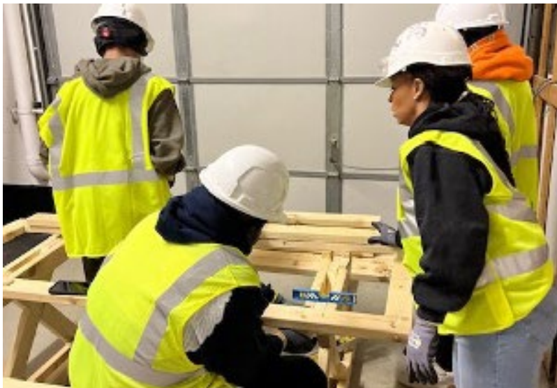
Photo, left: Youthbuild-EC crew members building picnic tables in the workshop.
