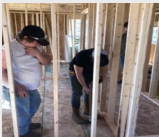
AEOA workshop building
